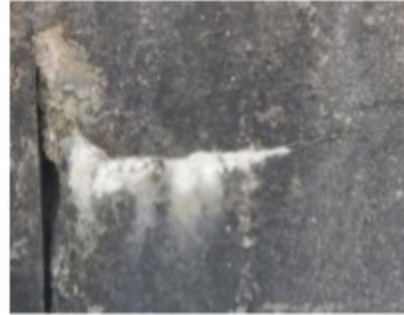
Efflorescences blanchâtres
